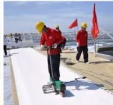
long side hot air welding
